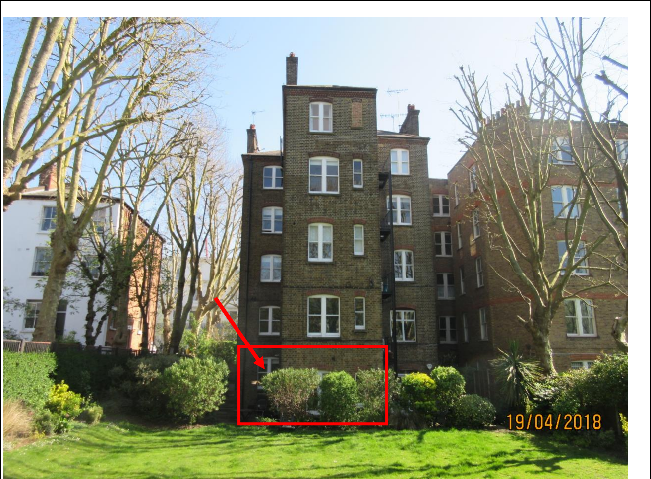
Rear elevation with Flat 2 outlined in red. Window to be altered indicated with an arrow
